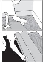
3. Apply a tackifier to the sub-floor using a roller, trowel or brush.
